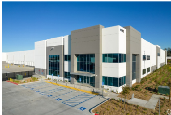
Typical Building Design with Concrete Wall Panels
